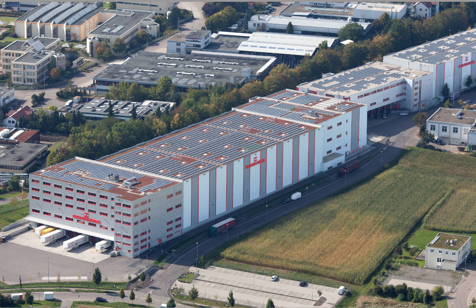
HELUKABEL® Headquarters Hemmingen/Stuttgart
