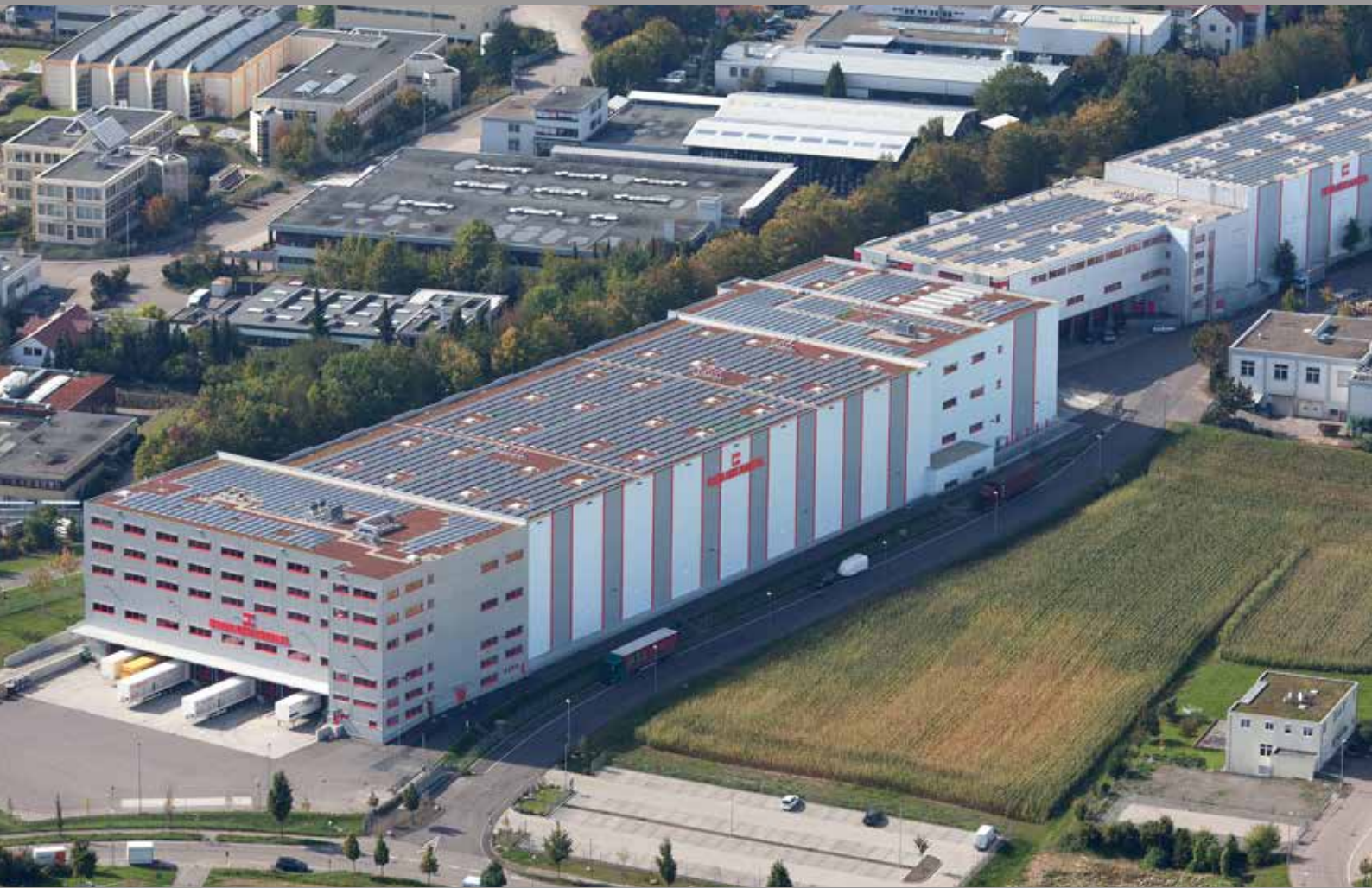
Logistics-Centre Hemmingen / Stuttgart
