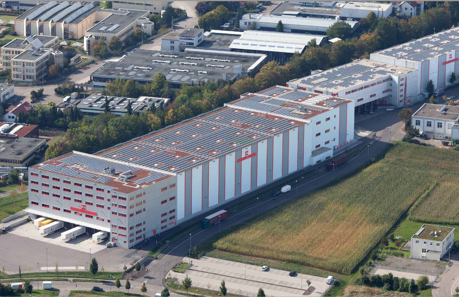
Logistics-Centre Hemmingen / Stuttgart
