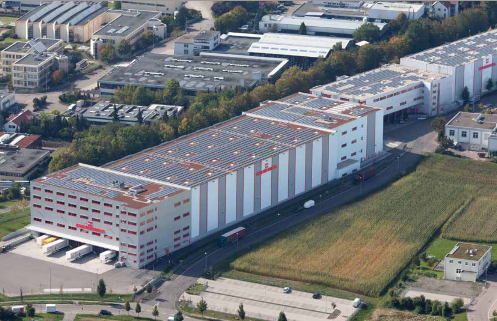
Logistics-Centre Hemmingen / Stuttgart
